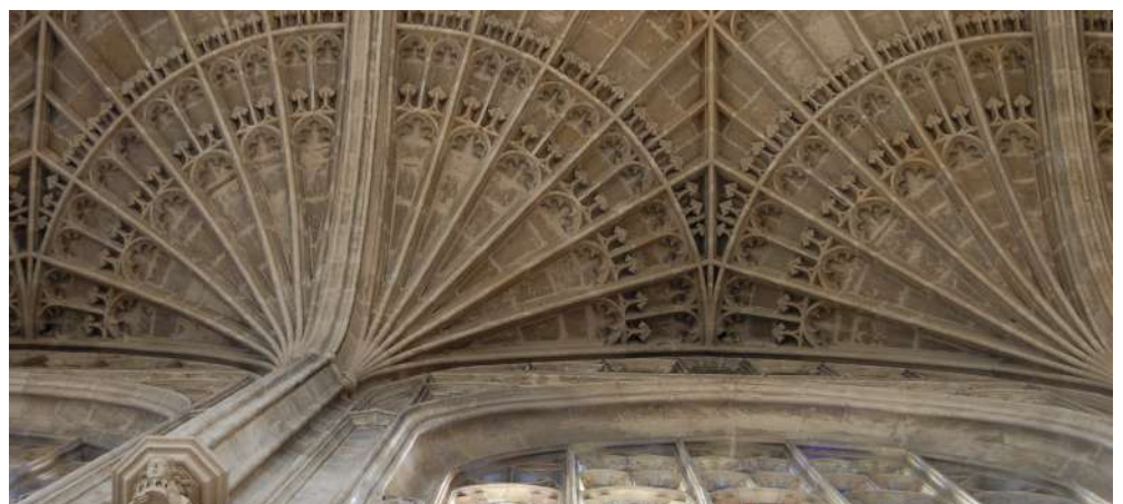
Fan Vaulting at King's College Chapel, Cambridge - Tom Ait and Creative Commons
